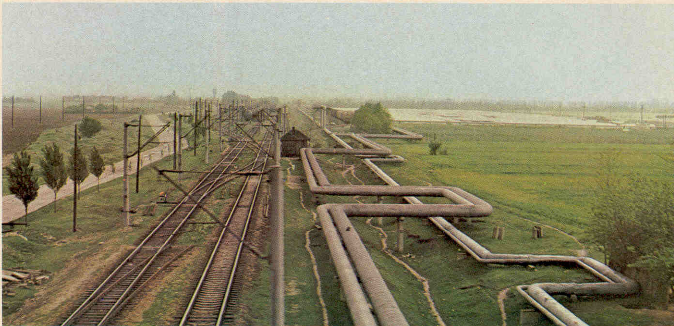
THE OIL FIELDS OF PLOESTI , about an hour's train ride north of Bucharest. Petroleum and petroleum products are key elements in Romania's growth-oriented economy.
